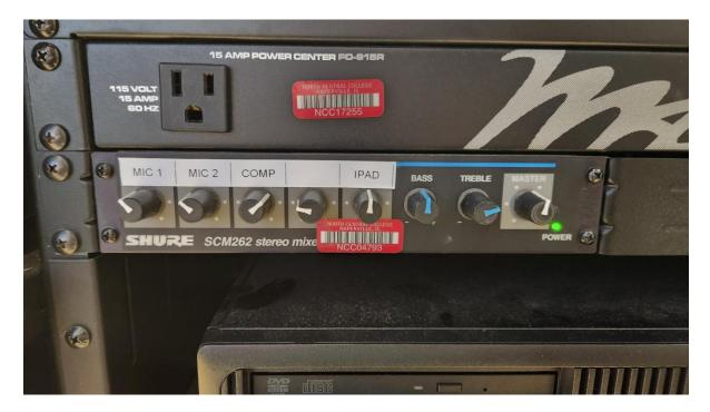
Turn the "COMP" knob to increase or decrease the volume of the computer audio going into the audio system. Make sure the "MASTER" knob is turned up as well. The "MASTER" knob adjusts all of the inputs equally, while the "COMP" know only adjusts the computer volume.
