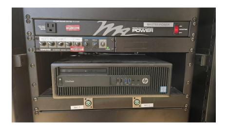
To begin, turn on the red main power switch located at the top right of the equipment rack.
